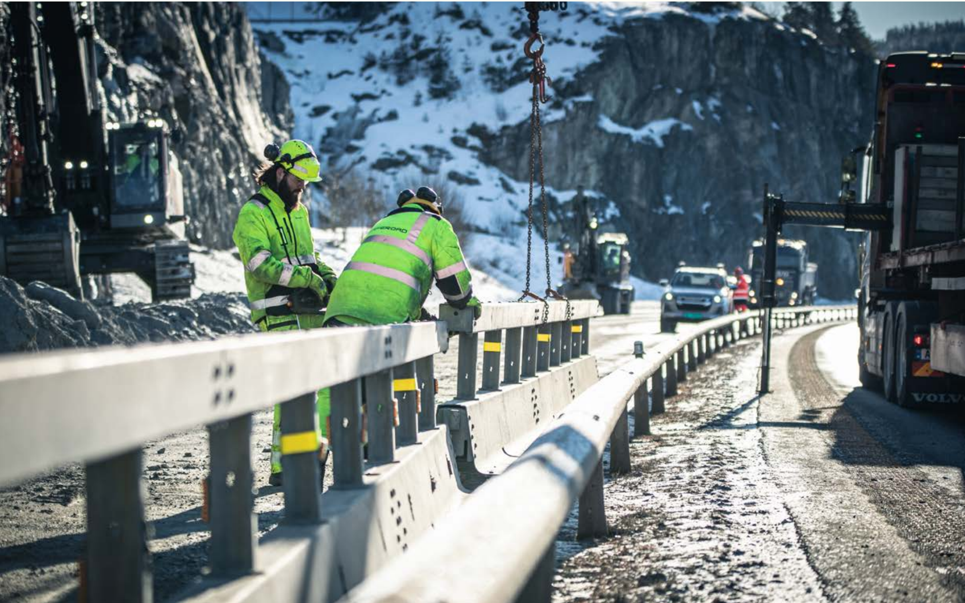
VarioGuard installation at European route E6 by Morskogen, Norway.
