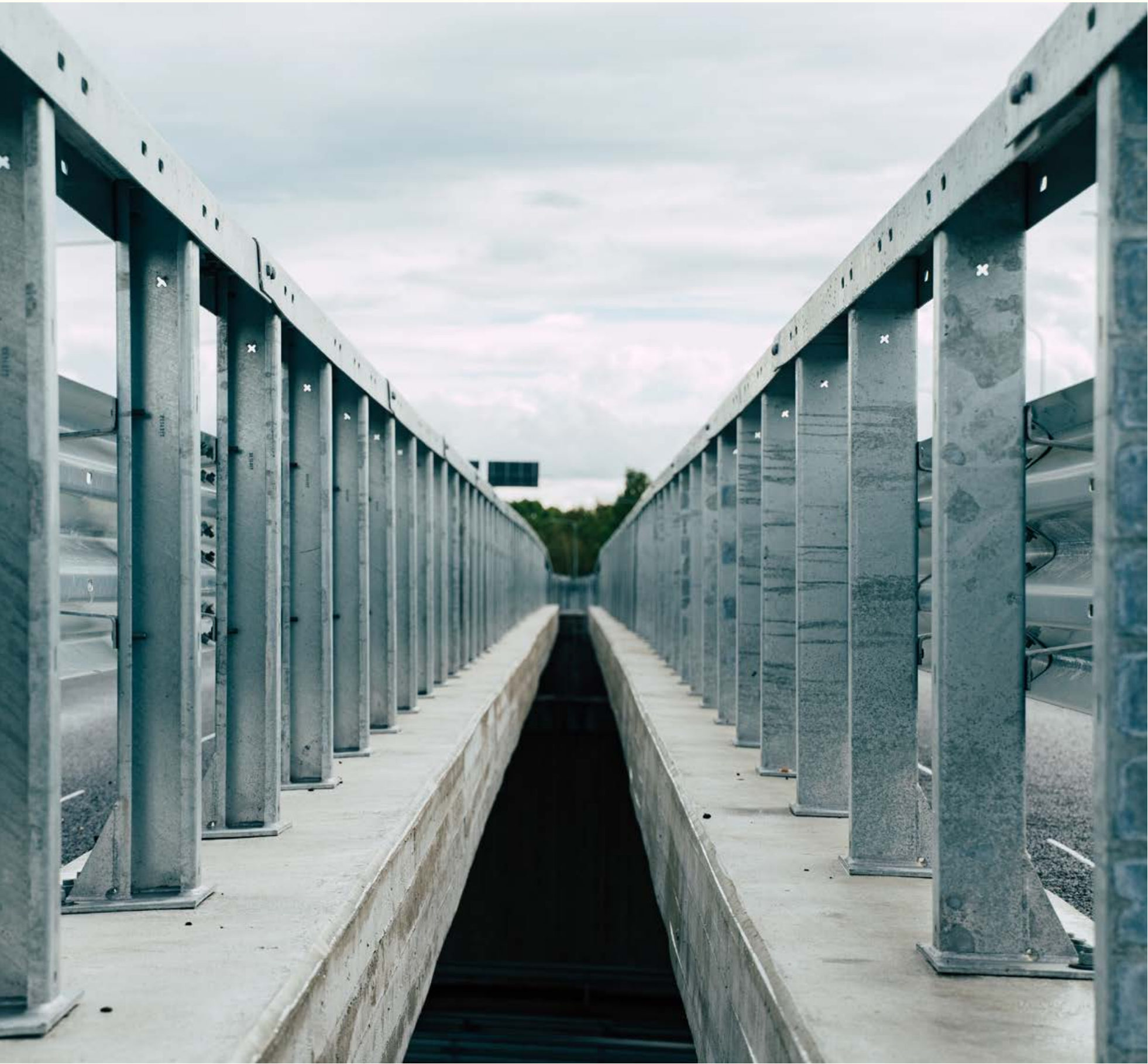
Our SafeStar and Megarail installed on the Tallinn-Pärnu highway. Project Kanama, Estonia.
